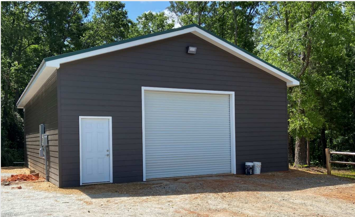
New Maintenance Building at Eilerslie Park (Constructed by Facilities Maintenance and Inmate Crews)
